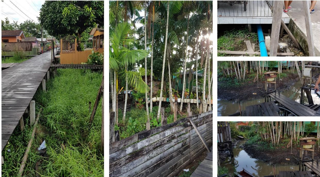
Figure 34.2 Infrastructure deficit in the city of Afuá, Pará, Brazil (Source: Laboratório de Estudo das Cidades Collection/UNIVAP).
