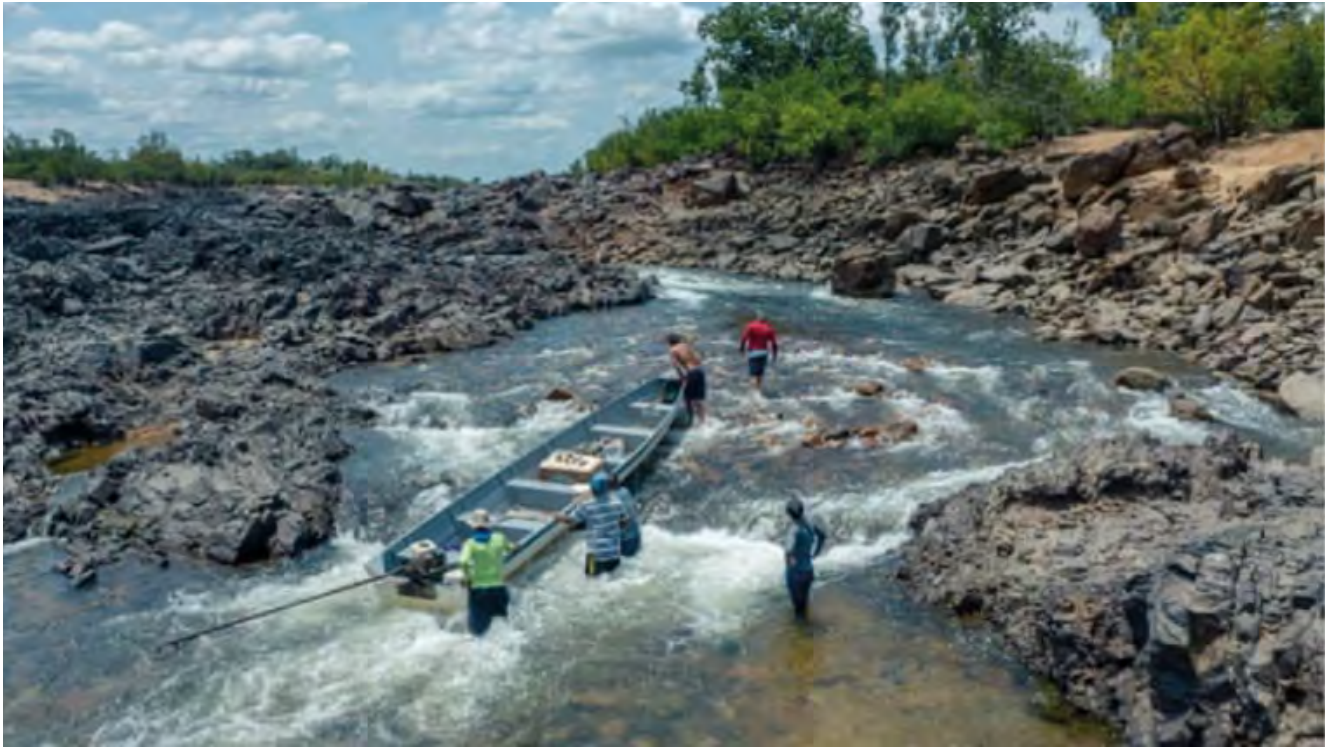
Figure 20.5 The Belo Monte hydroelectric project has diverted water from the “Volta Grande” (big bend) of the Xingu River, a 130-km stretch between the two dams that comprise the project. Source: Watts (2019). Photograph: Fábio Erdos/The Guardian.
